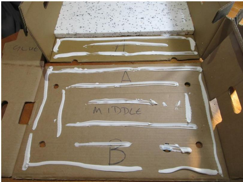
Gluing 2 boxes ready for installing the polystyrene sheet. When you install the polystyrene sheet, make sure you also run a bead of glue along the edge of the sheet where it adjoins the cardboard structure, for extra rigidity. Hold the sides more or less vertical with masking tape or string whilst the glue sets to help them stay upright.
